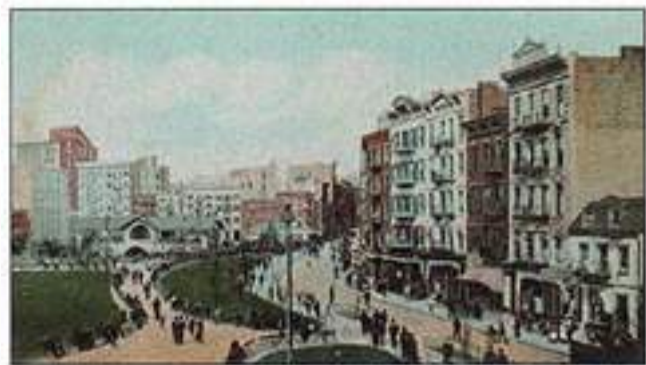
The Bandit's Roost and the first documented pizzeria in the US were demolished to build Mulberry Bend Park, now called Columbus Park.
